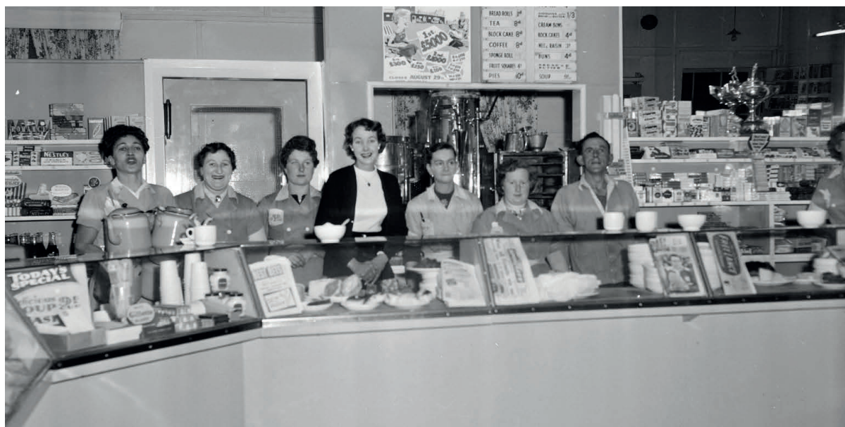
Refreshment rooms at Palmerston North Station 15 August 1959 - taken at 3 o'clock in the morning awaiting the arrival of 4 Special Rugby trains enroute to Wellington – Manawatu Evening Standard.
